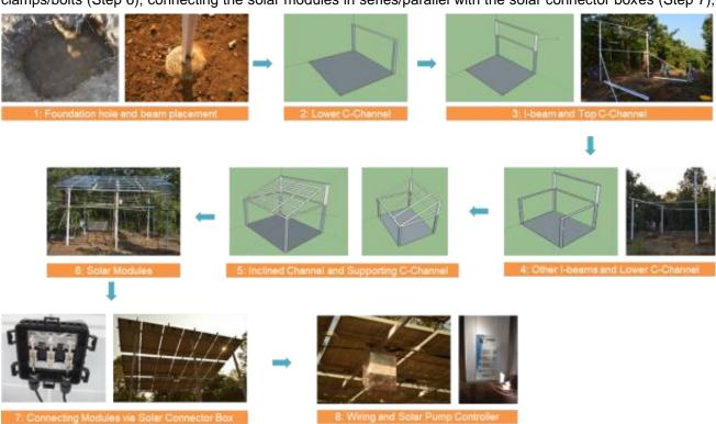
Figure 18: Pictorial representation of installation of SPIS
